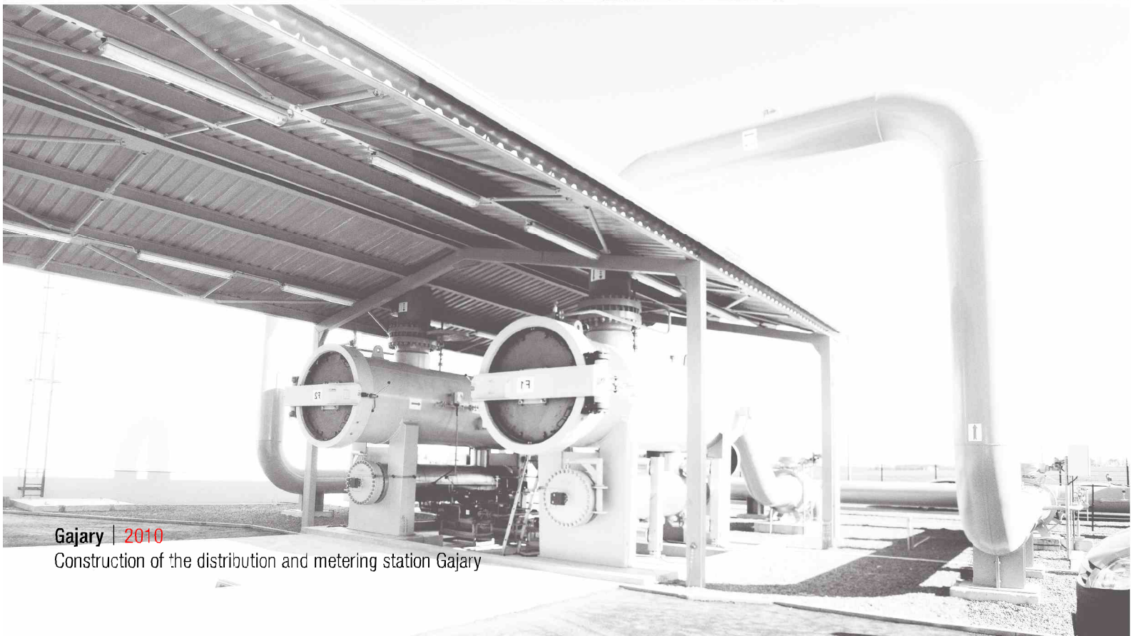
Gajary | 2010 Construction of the distribution and metering station Gajary
