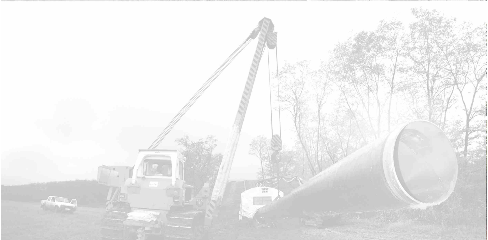
Nitra R1 | 2009 Erection of the pipeline – welding head group
