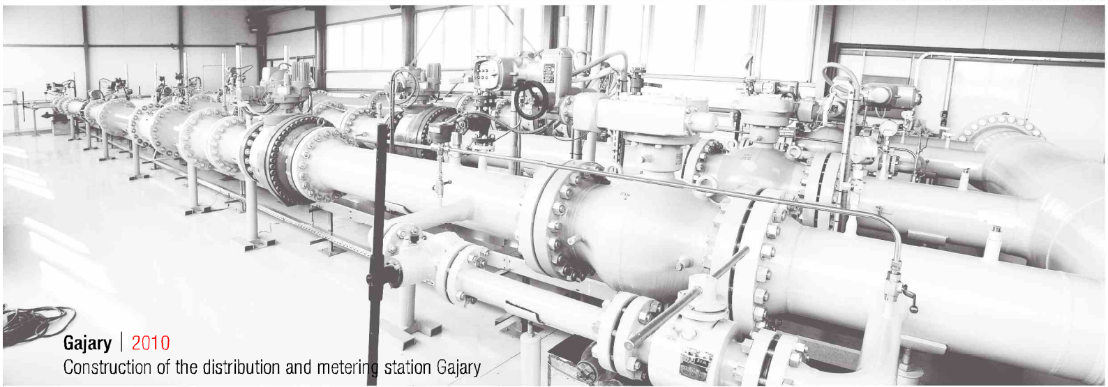
Gajary | 2010 Construction of the distribution and metering station Gajary
